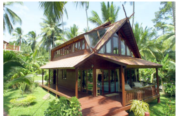
Figure 1.21: Traditional Village House of Malaya (Ford Foundation, 2001)
