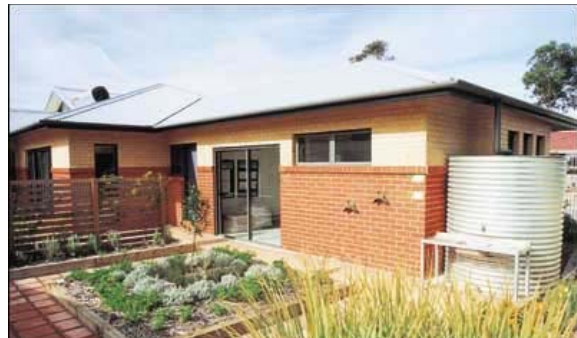
Figure 1.31: House on a Corner Site at Landcom's Melaleuca Estate at Metford (AGO, 2001)
